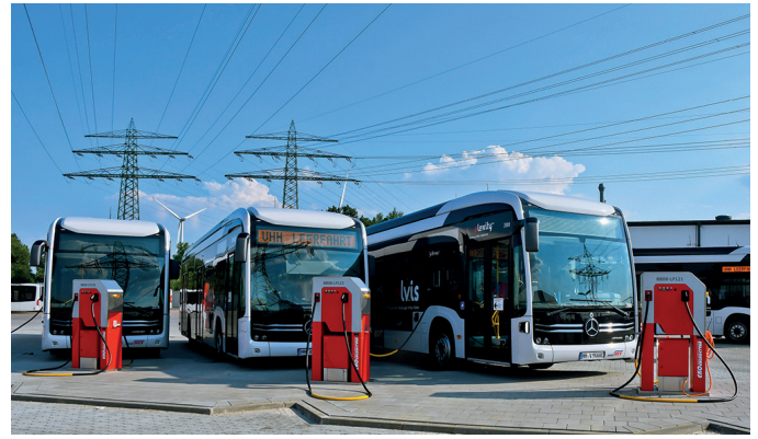
An intelligent charge management system ensures that all vehicles are charged as needed, cost-effectively and in a way that conserves batteries (© Ulrike Kabel/INIT)
